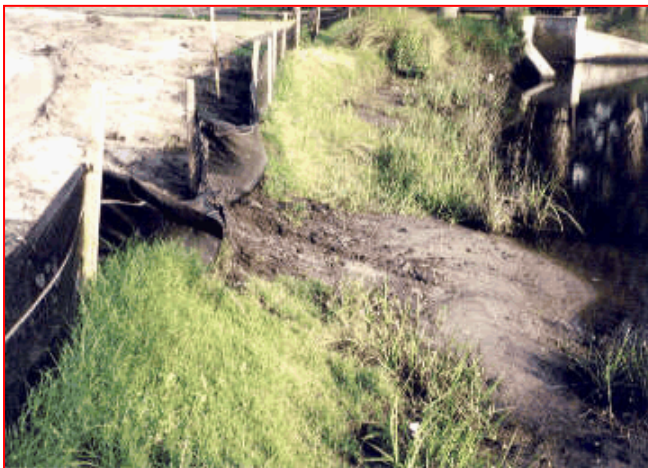
Don't. Install silt fence where flow velocity and volume will compromise structural integrity. If necessary, reinforce silt fence in sensitive areas.
