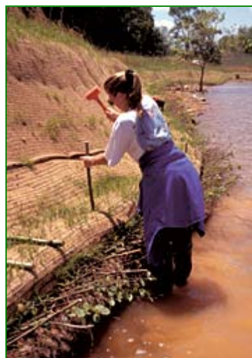
Do. Securely anchor the fiber roll to level contours with approved stakes.
