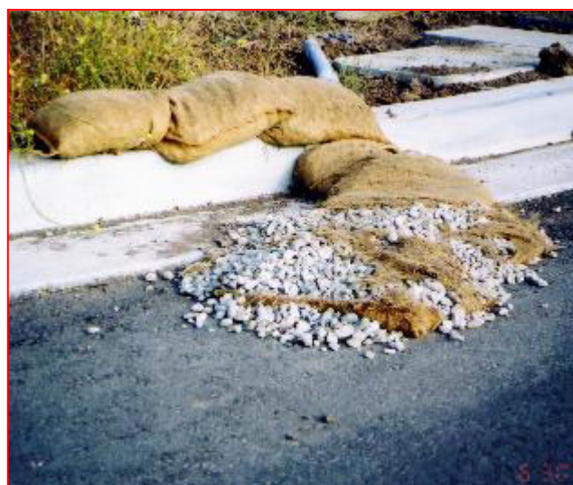
Don't. Allow bags to disintegrate and rupture spilling gravel. Gravel bag berms must be maintained to be an effective BMP.
