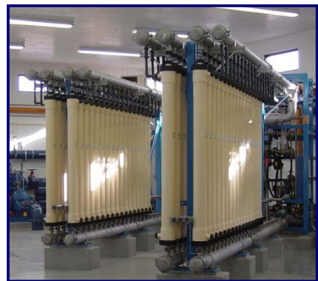
Figure 6-1: Membrane Filters
