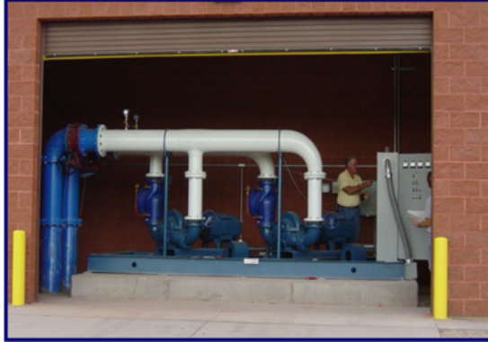
Figure 3-4: Treatment Plant Booster Pumps
