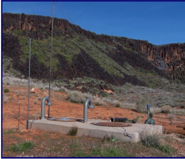
Figure 4-2: Air Release Lines
