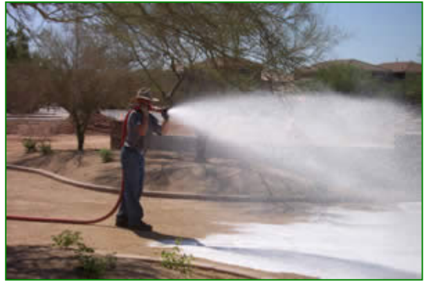
Do. Keep wind erosion low by applying water or other dust palliative when necessary.
