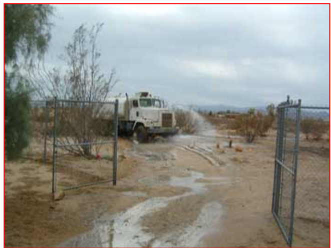
Don't. Apply so much water as to cause erosion from the runoff created.
