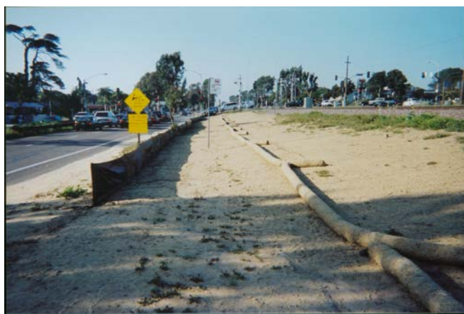
Do. Install fiber rolls with overlapping ends and place end where runoff will accumulate facing uphill.
