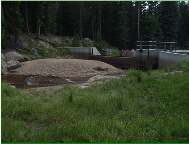
Do. Provide sediment trap for areas not large enough to require a sediment basin.
