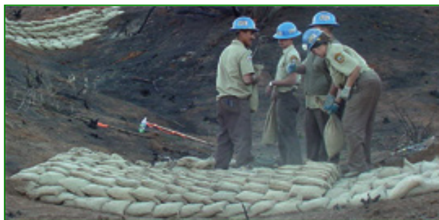
Do. Stack gravel bags with ends overlapping to create a diversion.
