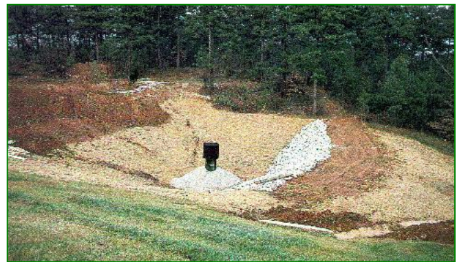
Do. Design an outlet structure that slows the flow to allow sediment to settle out of the runoff.
