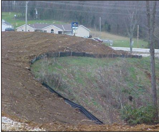
Do. Protect slopes from concentrated flows.
