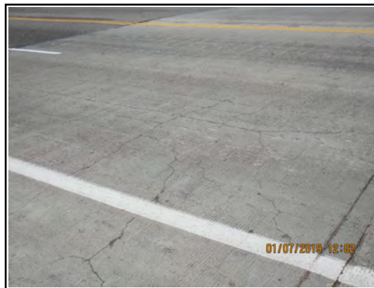
Approach Slab Map Cracks EBL Southwest
