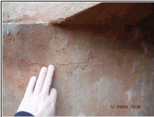
Center Wall Horizontal Cracking at W. End
