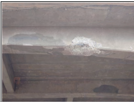
Girder 1 Span 2 Spall
