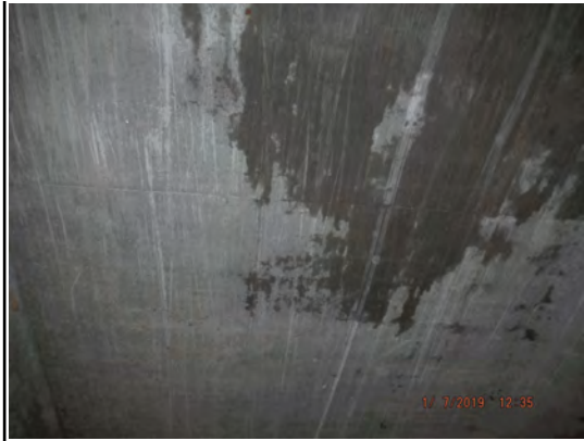
Top Slab Underside Scraping at Inlet of The N. Cell
