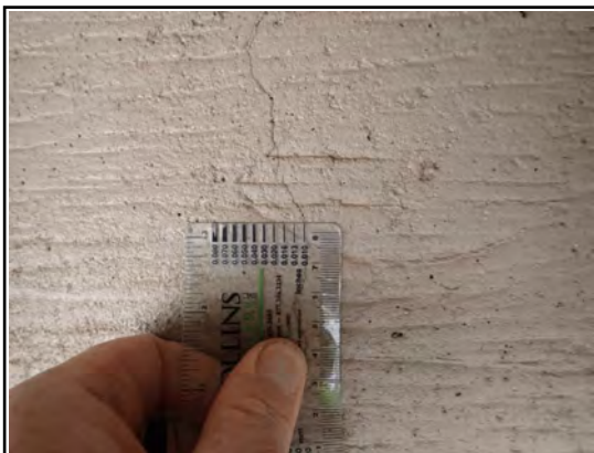
Abutment 1 Vertical Crack
