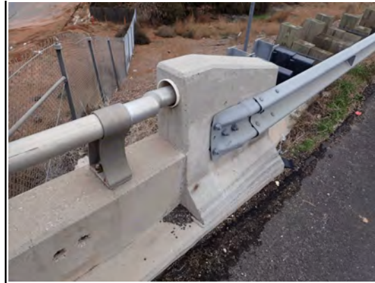
Parapet End Treatment
