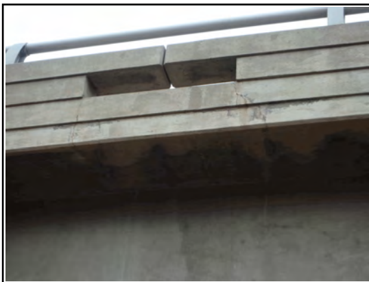
Parapet West Face Crack
