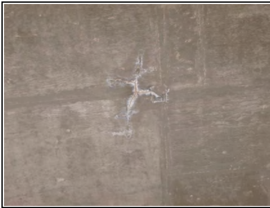
Deck Underside Span 3 Bay 3 Cracking
