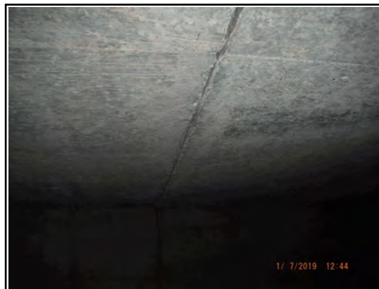
S. Cell Top Slab Underside W. Construction Joint
