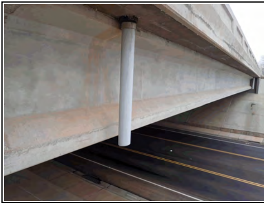
Typical Drain Pipe
