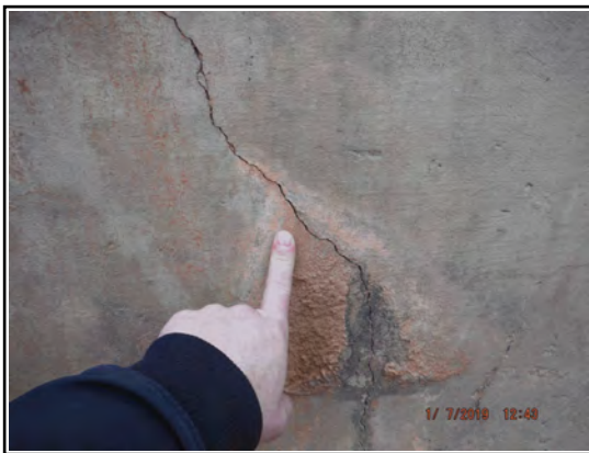
Wingwall S.W. Diagonal Cracking
