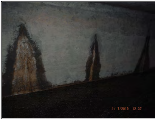
N. Cell Wall Vertical Cracking and Staining E. End
