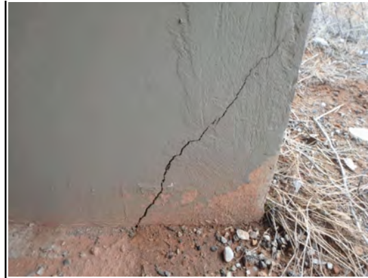
Abutment 1 Diagonal Crack
