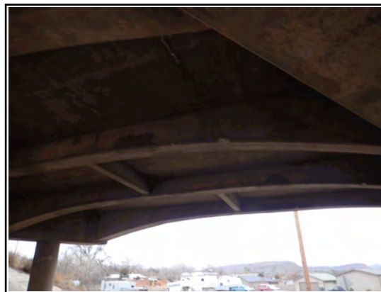
Girders 3 and 4 Span 2 Patches
