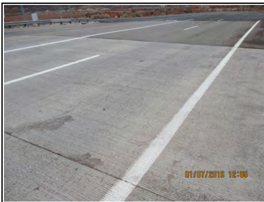
Approach Slab Map Cracks EBL Southeast
