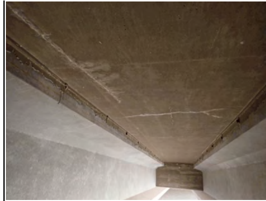
Deck Span 1 Bay 10 Longitudinal Cracking
