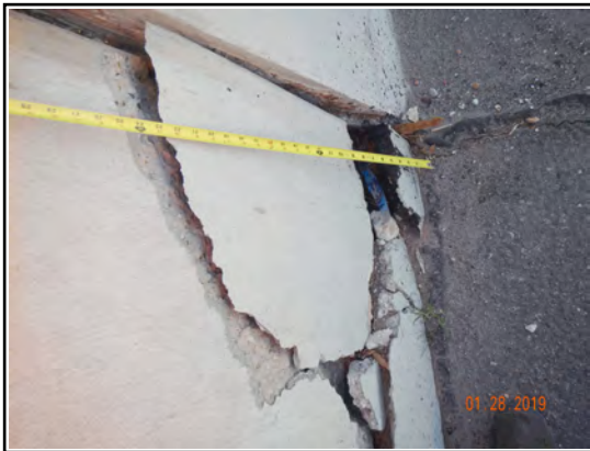
NE Corner Approach Barrier Spall
