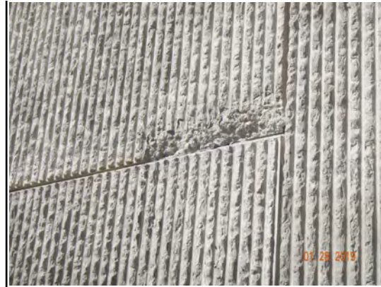
MSE Panel Spall @ NE Corner
