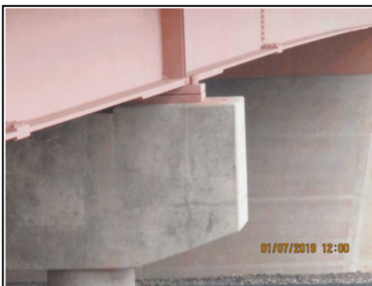
Bearing Fixed Girder 7 Bent 2
