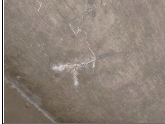
Deck Underside Span 3 Bay 2 Cracking
