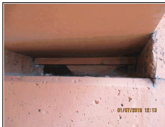
Bearing Fixed Girder 7 Abutment 2
