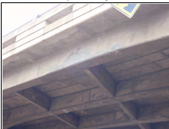
Girder 5 Span 2 Patch
