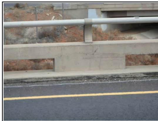
South Parapet Cracking
