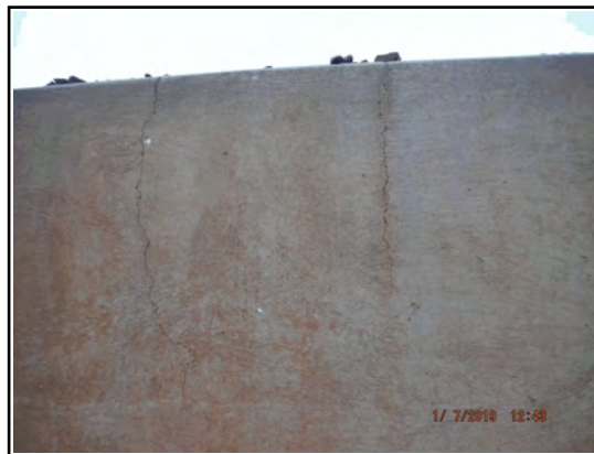
W. Headwall Vertical Cracking
