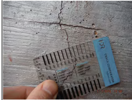
N. Cell Wall Vertical Cracking
