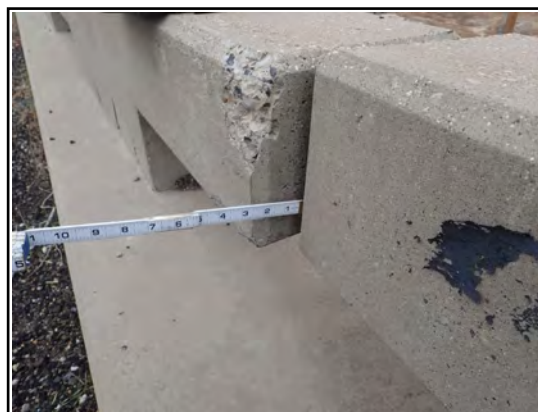
East Parapet Distortion Damage
