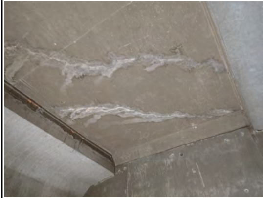
Deck Span 1 Bay 5 Diagonal Cracking
