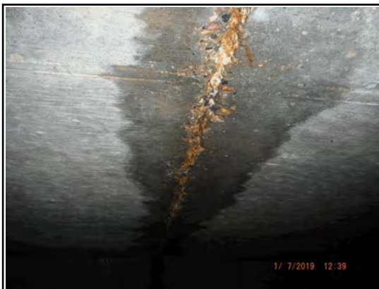
N. Cell Top Slab Underside Center Construction Joint
