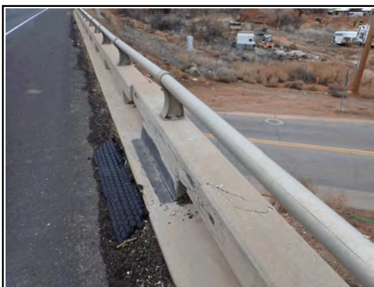
East Parapet Distortion
