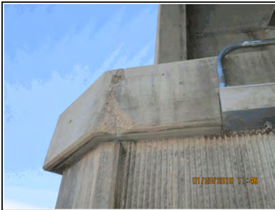
MSE Wall Spall Northwest Coping
