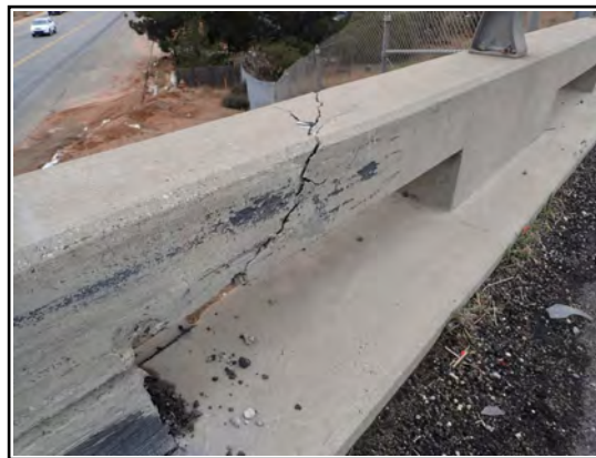
East Parapet Cracking
