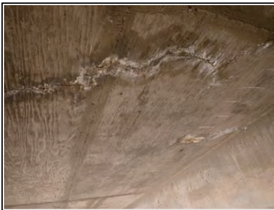
Deck Span 1 Underside Bay 2 Cracking
