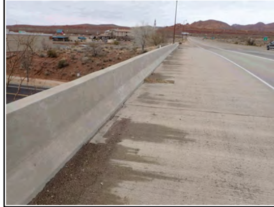
Typical Parapet and Shoulder
