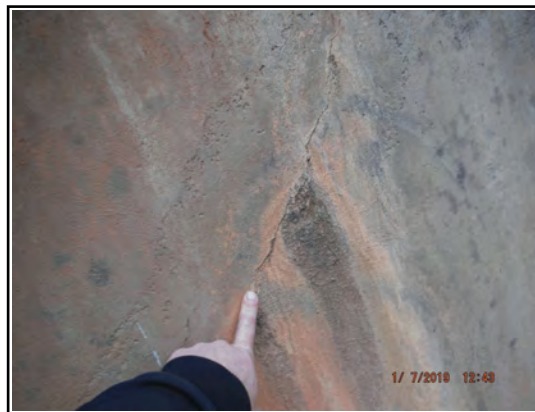
Wingwall N.W. Diagonal Cracking
