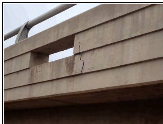
Exterior Parapet Span 3 Delamination
