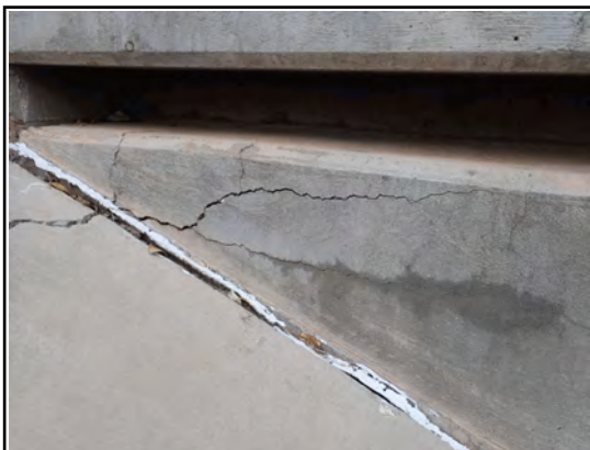
Southwest Wingwall Crack
