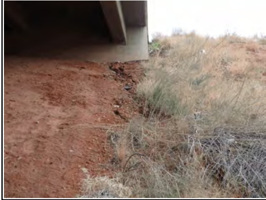
Southwest Slope Erosion
