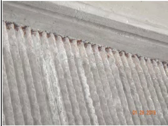
MSE Panel Cracking @ Abutment 2 W. Corner
