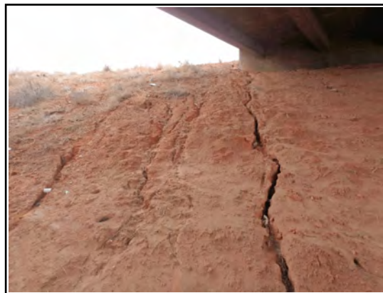
Northwest Slope Erosion
