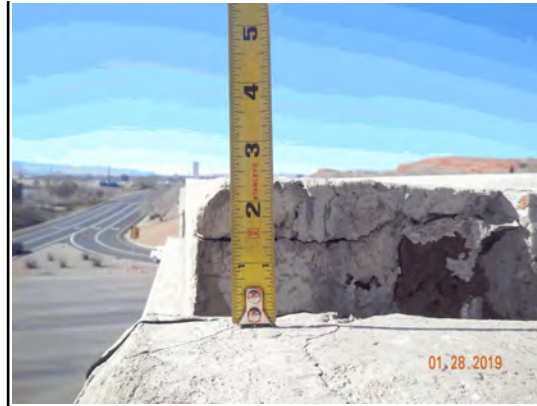
NE Corner Approach Barrier Settlement
