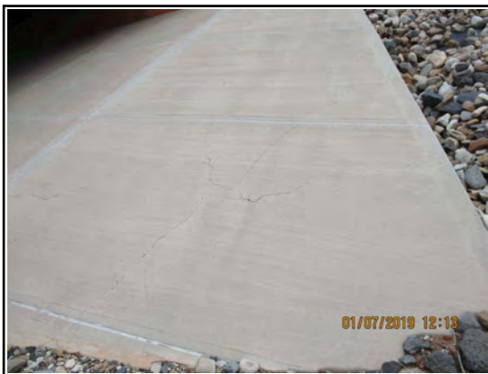
Concrete Slope Protection Cracks Southeast
