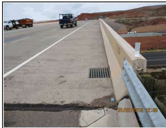
Approach Slab Drain From Northeast
