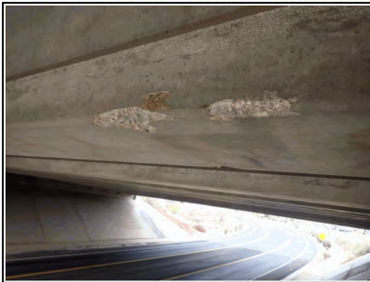
Girder 13 Near Abutment 2 Spall
