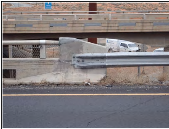
Northwest Guard Rail Connection with Missing Bolts
