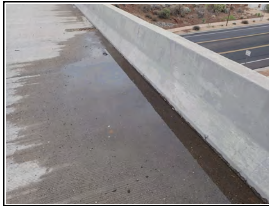
Ponding at Southeast Approach
