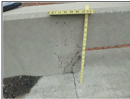
West Parapet Delamination
