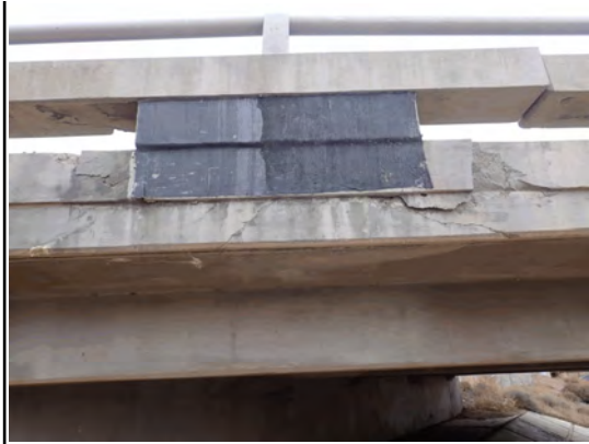
East Parapet Span 1 Exterior Patch
