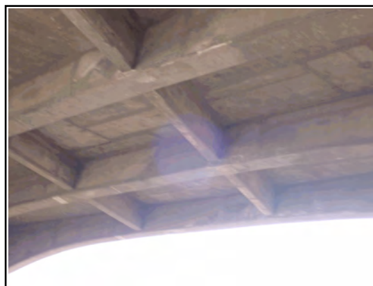
Girders 1-3 Span 2 Patches
