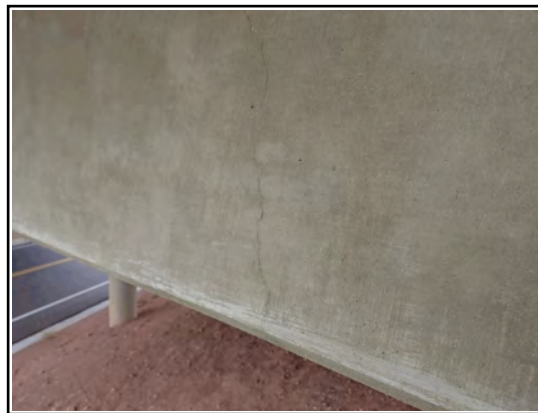
Girder 4 Span 3 Cracking
