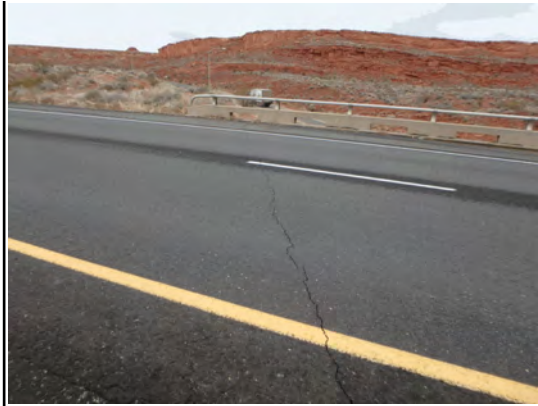
Backwall Joint Crack
