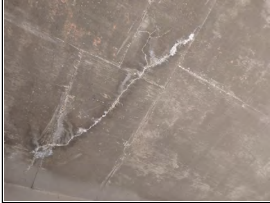
Deck Underside Span 1 Bay 4 Cracking
