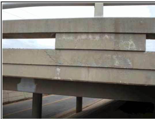
Parapet North Face Cracking
