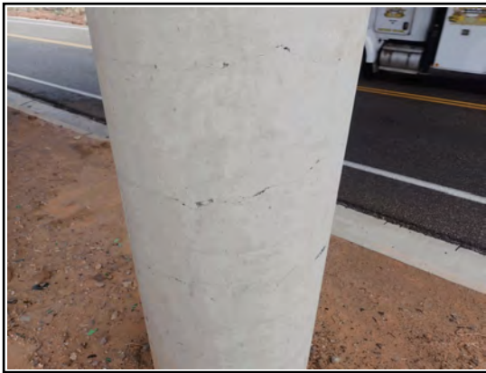
Bent 3 Column 1 Horizontal Cracking
