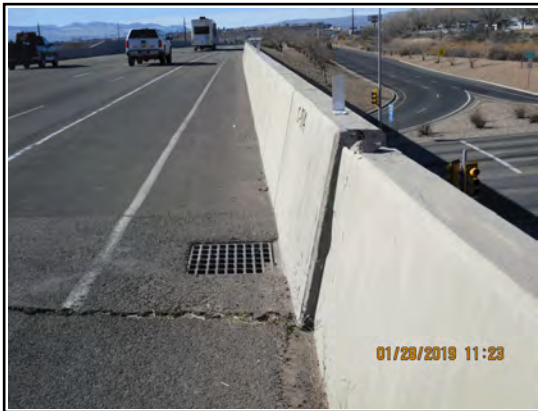
Approach Slab Drain Northwest
