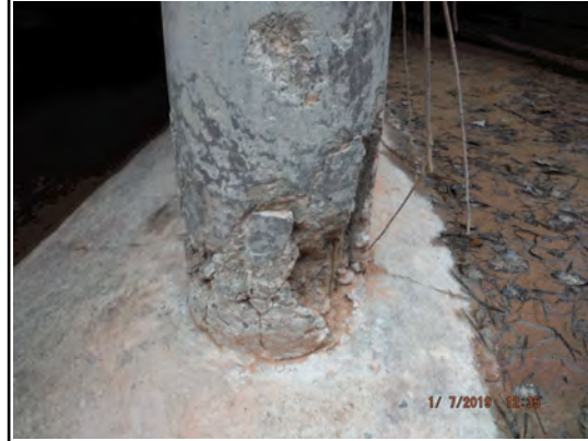
Center Wall Spall at Inlet
