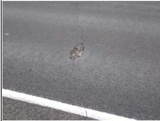
Lane 2 Pothole at South Relief Joint
