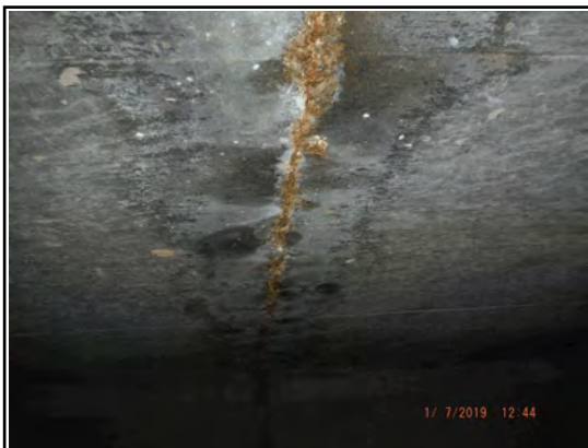
S. Cell Top Slab Underside Center Construction Joint
