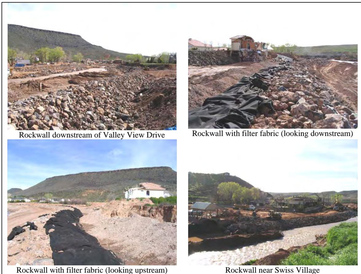
**Figure 24. Ground photos of the NRCS rock wall construction**
